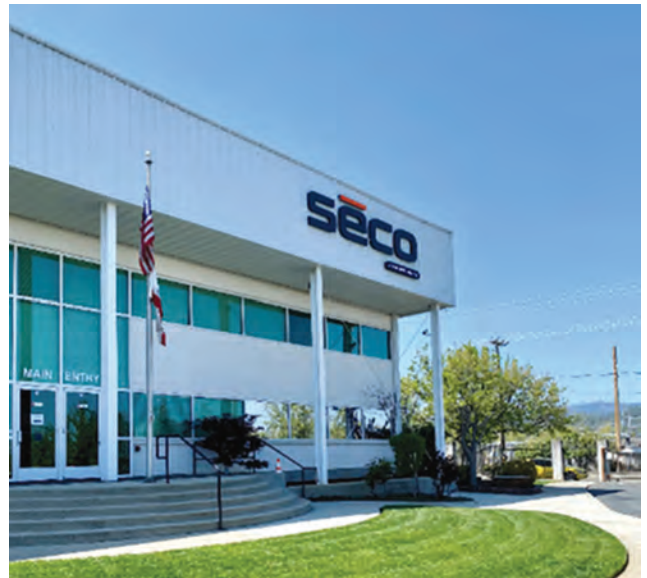
The SECO facilities at Redding, CA.
